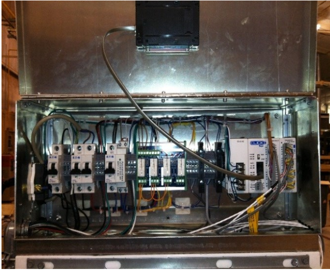
a) PLC Control/Monitoring Box—Internal
