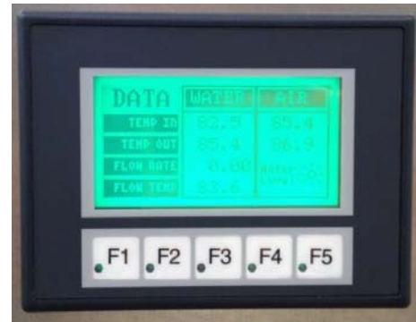
e) Temperature Setpoint Control Screen
