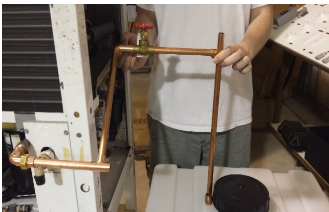
c) Piping Installation and Testing
